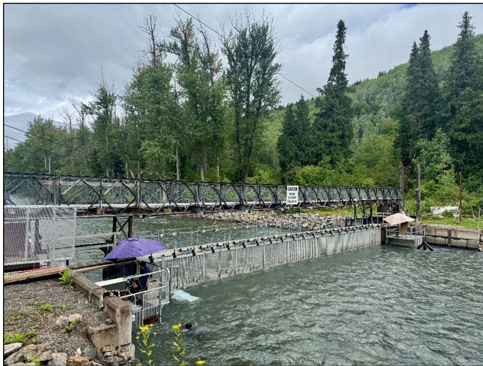
Downstream view of KSEF on July 31, 2026
