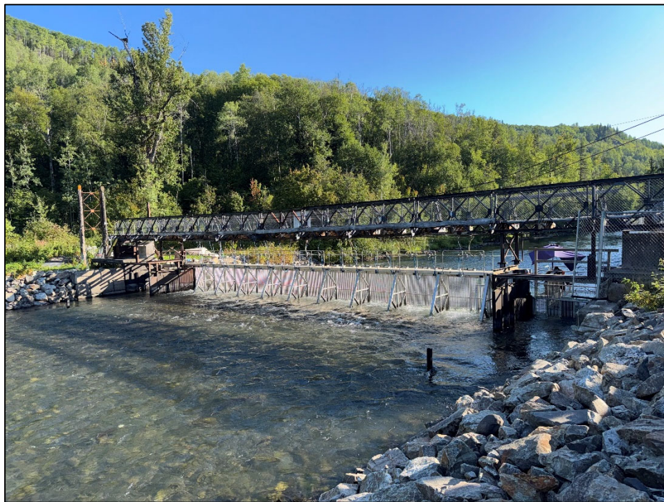
Upstream view towards the right bank at KSEF on August 14, 2026
