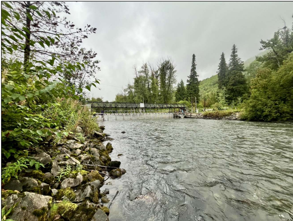
View downstream at the KSEF on August 28, 2026
