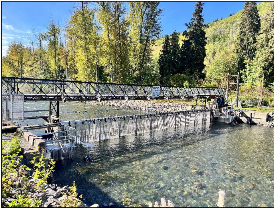
View downstream at the KSEF on September 17, 2026
