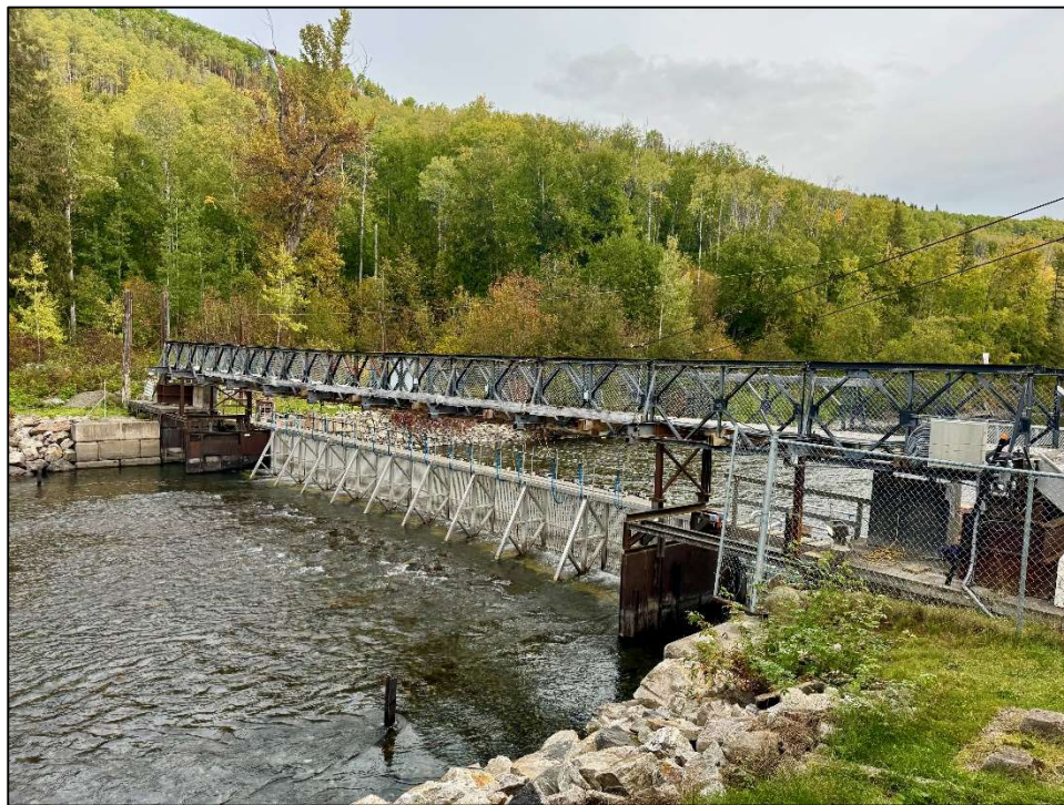
View upstream towards right bank at the KSEF on September 25, 2026
