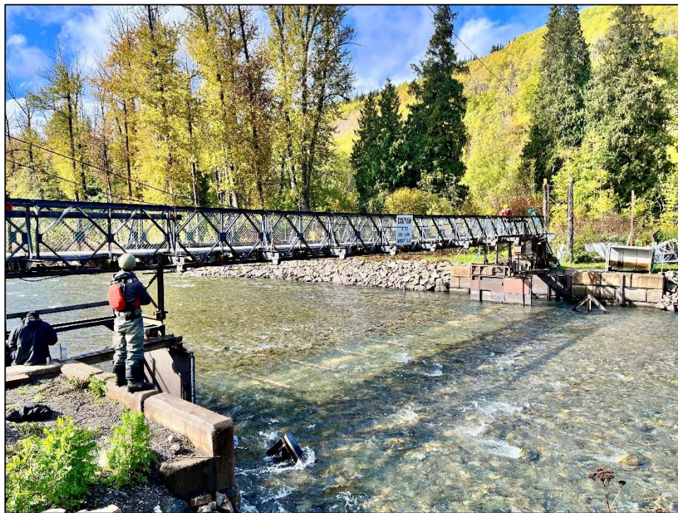
View downstream of fence removed on September 28, 2026
